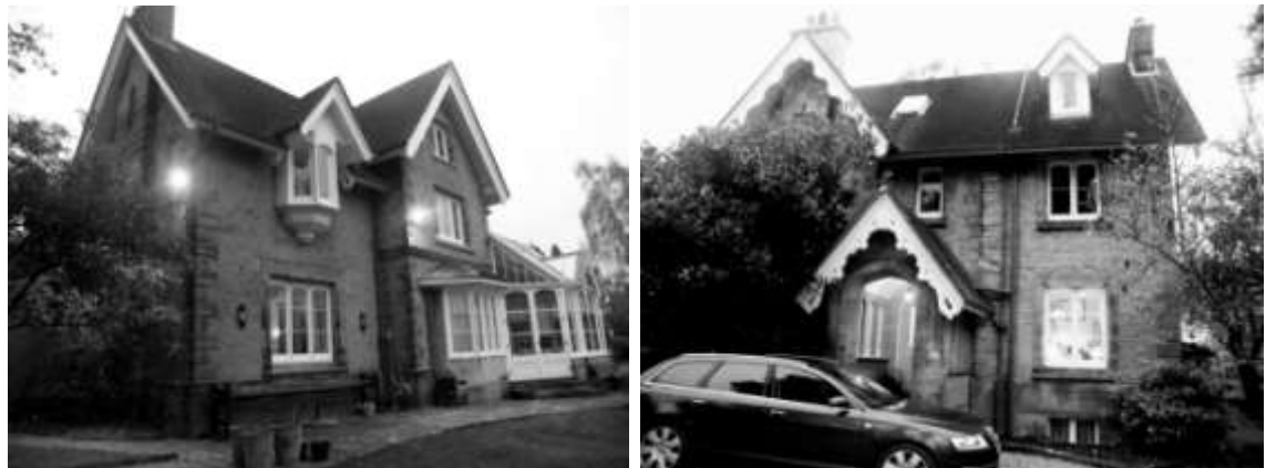
Figure 42. Calverley Park, no. 3. Left: garden front. Right: entrance front. Source: author.
